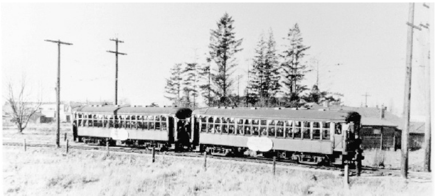
Photograph of the interurban tram leaving Steveston on its last run. City of Richmond Archives 1978 21 32.
