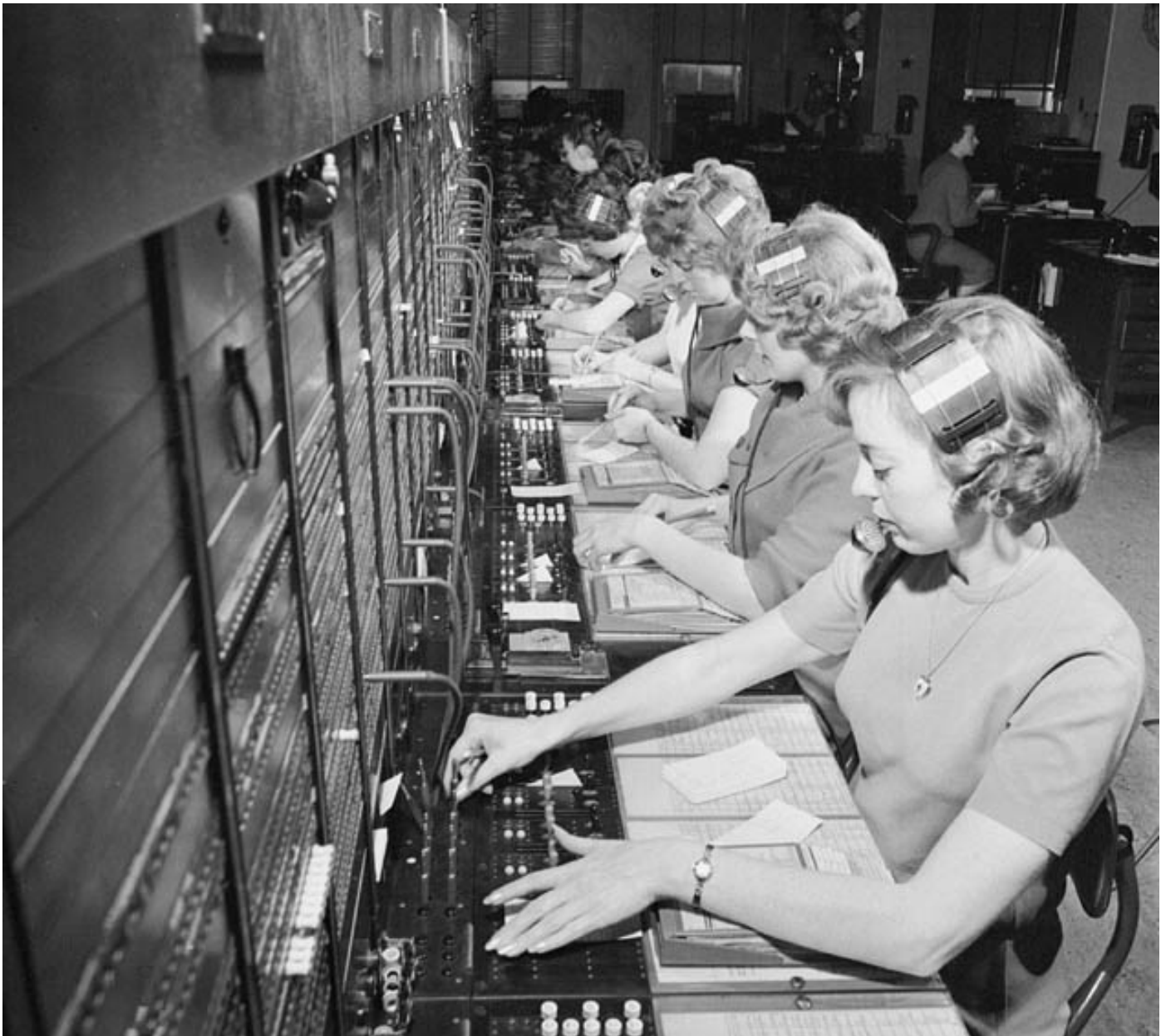
Long-distance switchboard at Bell Telephone Co., 1961.
